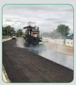
Application of aggregates and prime coat
