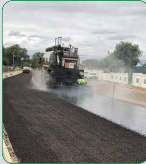
*Application of aggregates and prime coat*
