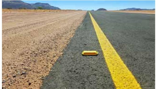
*Low volume sealed road with road markings and cat eye reflectors*
