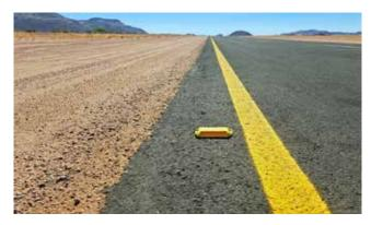
Low volume sealed road with road markings and cat eye reflectors
