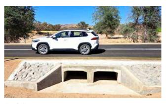
Twyfelfontein low volume sealed road showing the highquality drainage structure
